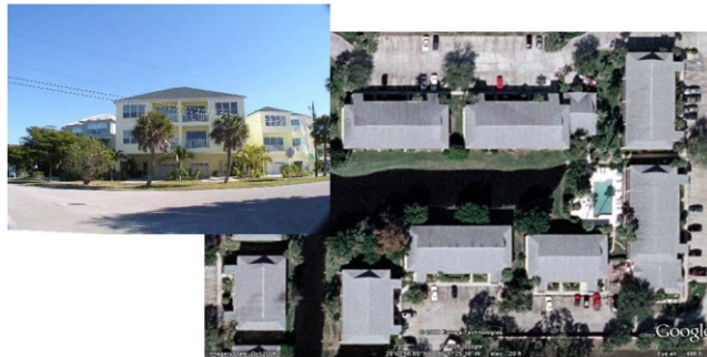
Figure 11. Typical low-rise buildings (LR).
