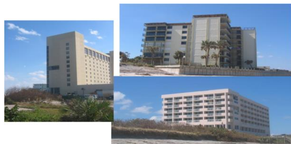
Figure 14. Examples of mid- and high-rise buildings (MHB).
