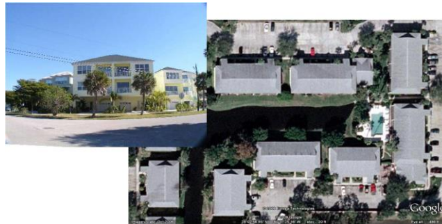
Figure 13. Typical low-rise buildings (LB).
