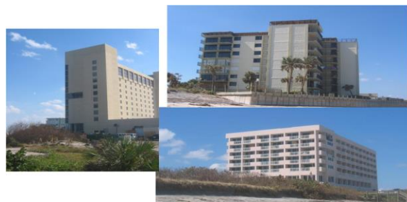
Figure 14. Examples of mid- and high-rise buildings (MHB).
