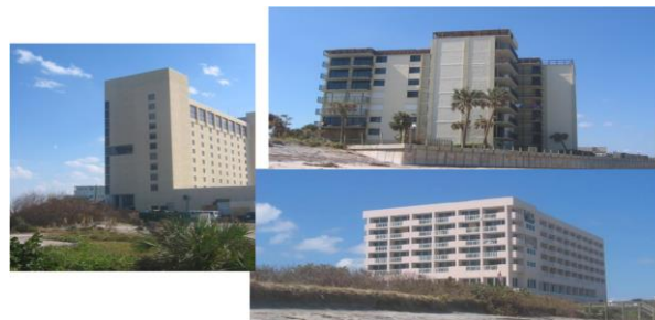
Figure 14. Examples of mid- and high-rise buildings (MHB).
