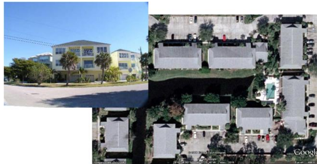
Figure 13. Typical low-rise buildings (LB).
