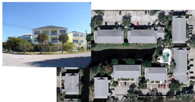
Figure 13. Typical low-rise buildings (LB).
