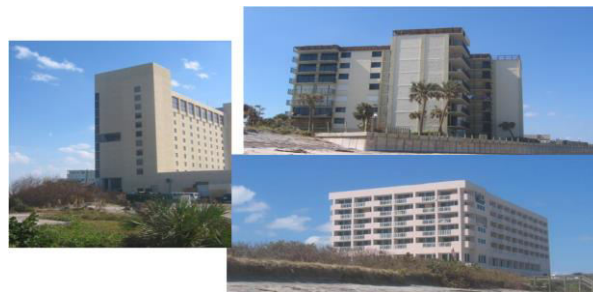
Figure 14. Examples of mid- and high-rise buildings (MHB).
