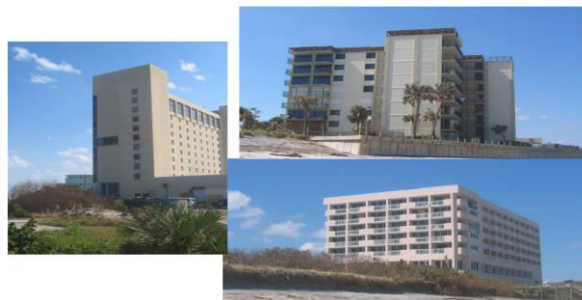
Figure 14. Examples of mid- and high-rise buildings (MHB).
