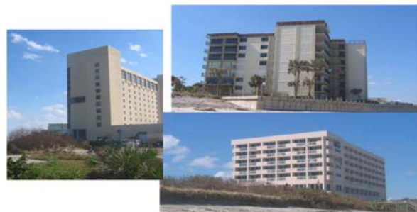
Figure 14. Examples of mid- and high-rise buildings (MHB).
