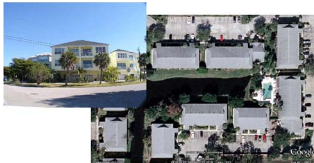
Figure 13. Typical low-rise buildings (LB).
