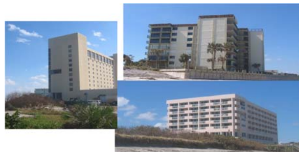
Figure 14. Examples of mid- and high-rise buildings (MHB).
