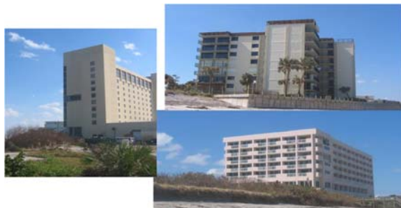
Figure 14. Examples of mid- and high-rise buildings (MHB).
