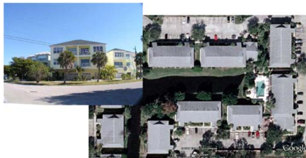
Figure 13. Typical low-rise buildings (LB).
