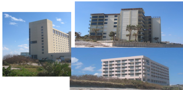
Figure 14. Examples of mid- and high-rise buildings (MHB).
