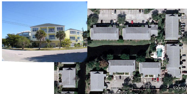
Figure 13. Typical low-rise buildings (LB).
