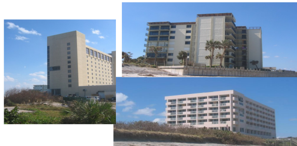
Figure 14. Examples of mid- and high-rise buildings (MHB).
