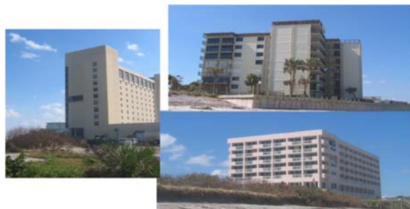
Figure 14. Examples of mid- and high-rise buildings (MHB).
